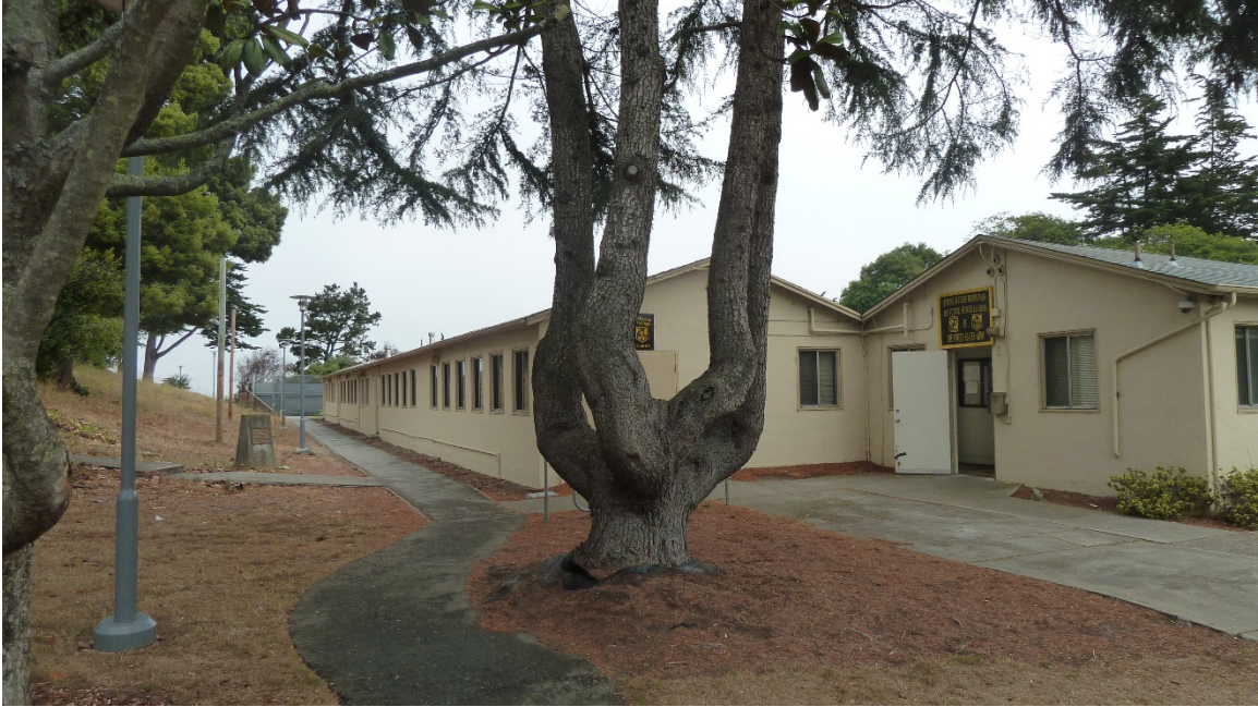
Figure 41: Underhill Building (future student residence hall location) looking north towards the tennis courts
